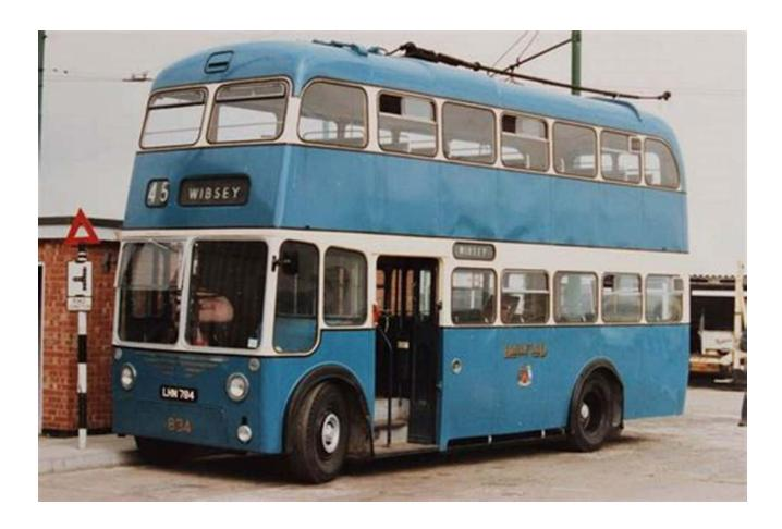
Bradford's embrace of trolleybuses can be traced back to the early 20th century when the city was experiencing rapid industrial growth. Unlike traditional tramways that required expensive infrastructure, trolleybuses offered a more flexible and cost-effective alternative. They were powered by overhead wires, which provided electricity to the buses through two poles attached to their roof.
